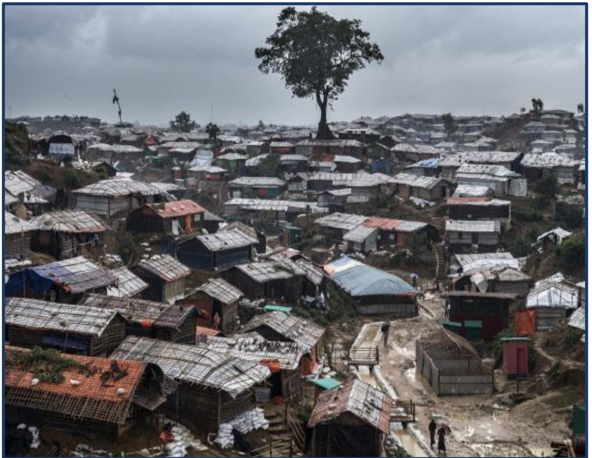
Figure: 2 - Camp 2: Overcrowded shelters at Rohingya Refugee camp in Cox's Bazar.
